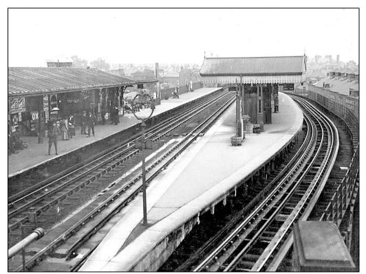
**Left:** Insofar as Putney Bridge was concerned, the Down platform was converted into a bay platform and a new third platform added was ʻaround the back' through widening. The third track became operational from 24 April 1910 with the completion of the project two months later. This view looks east from the westbound (Down) side. From 12 January 1911 the buffer stop in the new bay platform was replaced by oil resistance buffer, its outer end just visible at lower left.
